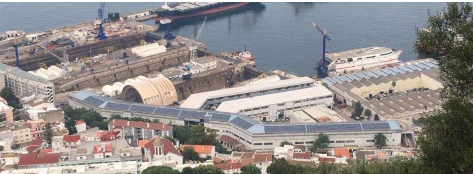
Figure 12. Solar panel array at New Harbours
