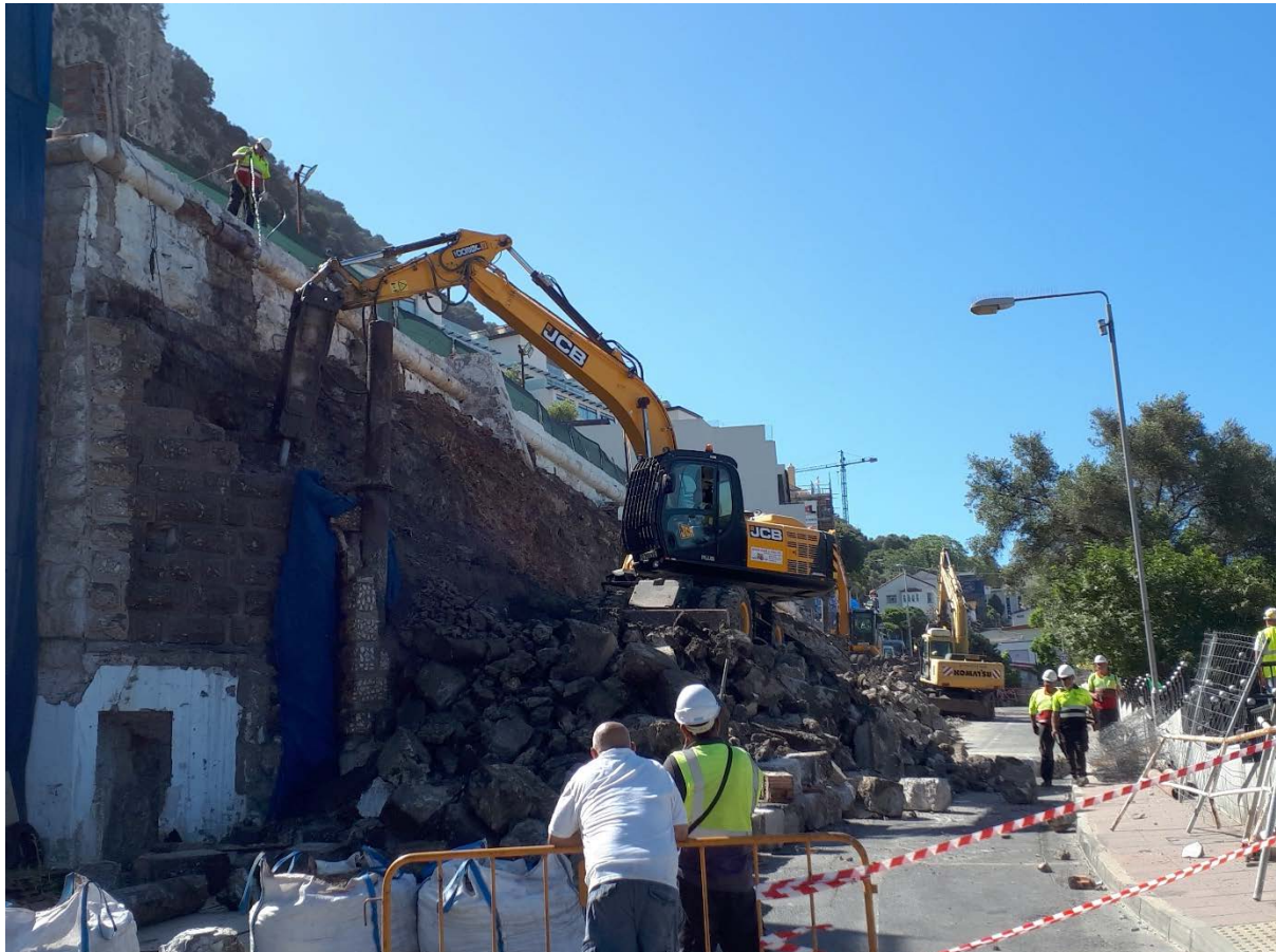
Demolition of the late 19 th -century blast wall erected originally to protect the two huge historic water tanks on Europa Road in August 2021. The demolition was monitored by archaeologists from the Gibraltar National Museum, funded by the developer. The tanks themselves are to be preserved within The Reserve residential development and the demolition revealed the original limestone façade. The development will also re-use material from the catch pits in an iconic entrance and include information on the site's history for residents and visitors.
