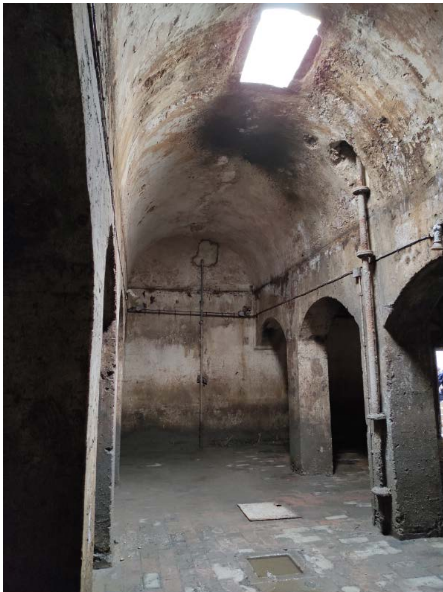
Nun's Well, Europa Flats, now open to the public. An underground reservoir thought to date to the medieval, Moorish period, though it may be earlier; it is the earliest structure linked to water supply in Gibraltar. Its interior is whitewashed with lime.
