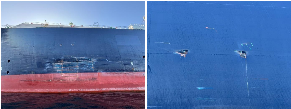
Figure 4 - General View of Port side hull damage & breached / holed hull
