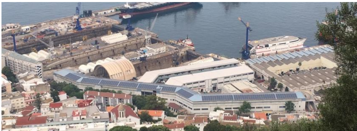
Figure 12. Solar panel array at New Harbours
