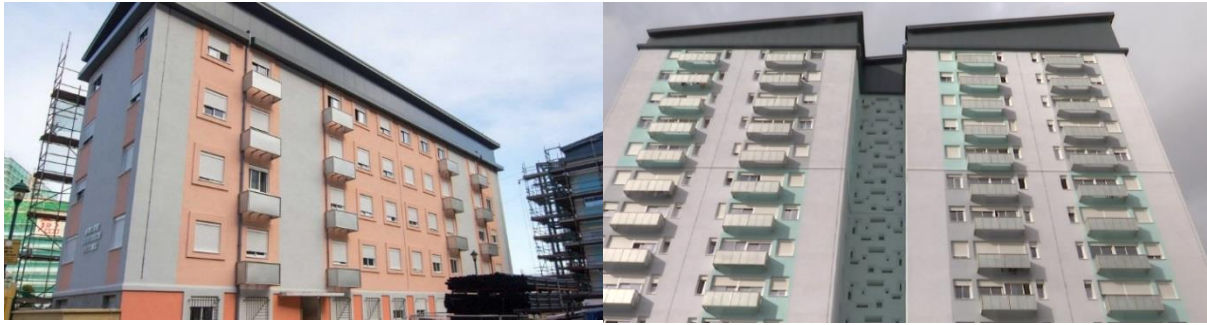
Figures 9. Refurbishment works at Laguna and Glacis Estates
