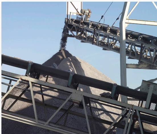
CONCRETE BATCHING PLANT
