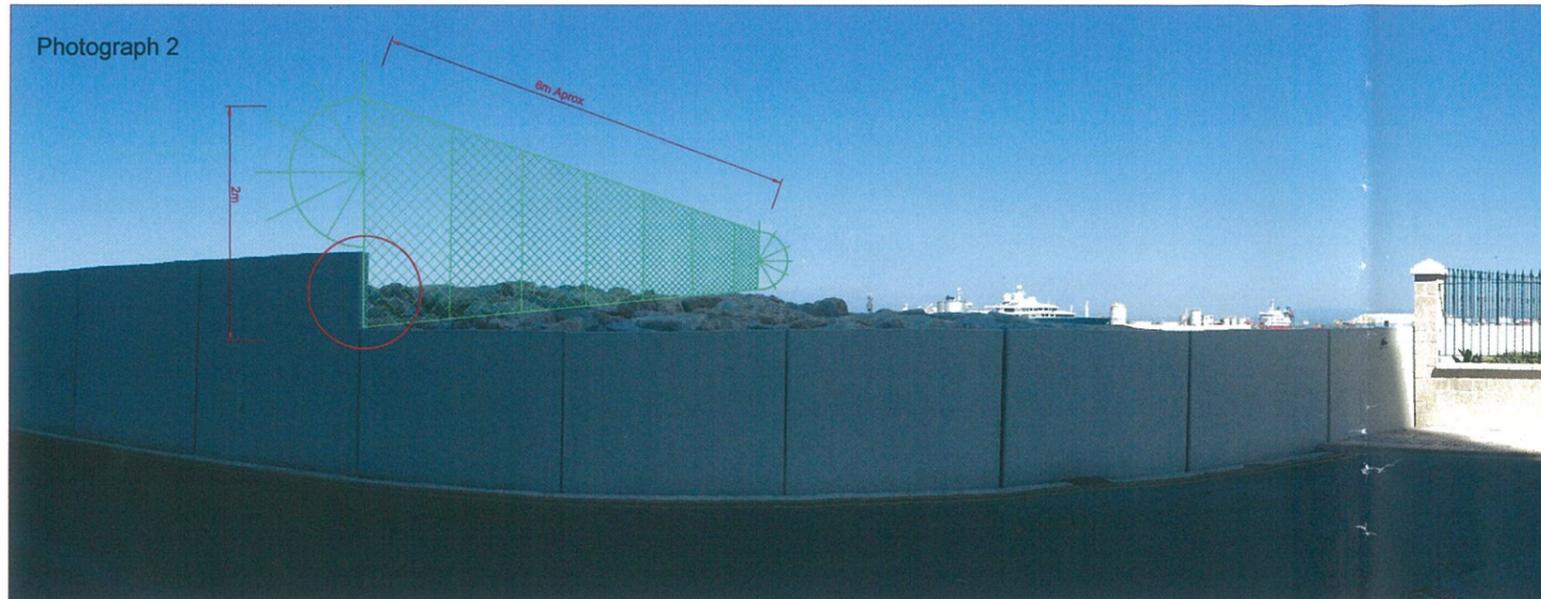
Figure 2 - Fencing with fan setup to be installed along the width of the revetment on the park side (North End).
