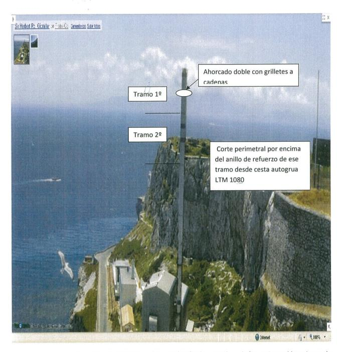
Once inspected and confirmed the first 2 lengths of the stack is firmly secured, ready for cutting and lowering to the ground, 2 operators will be hoisted in the metal basket attached to the LTM-1080; equipped with oxy settling cutting equipment will proceed to cut right round the stack just above the joint of the second length of chimney and the attached access ladder.
