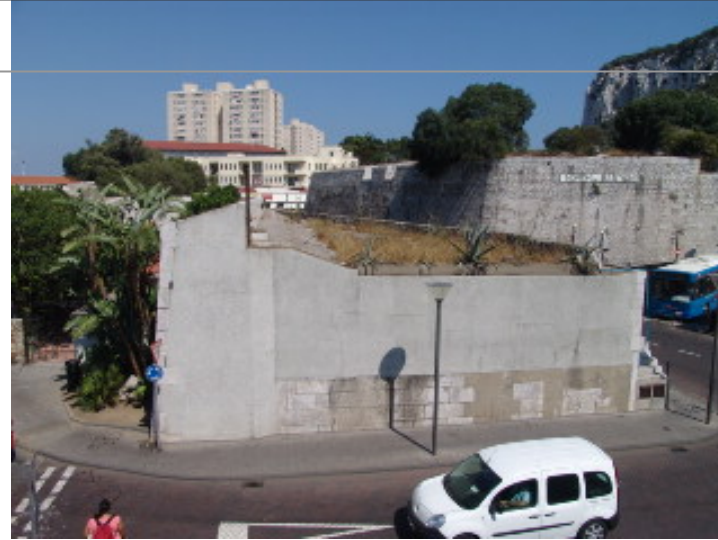
North Bastion Counterguard
