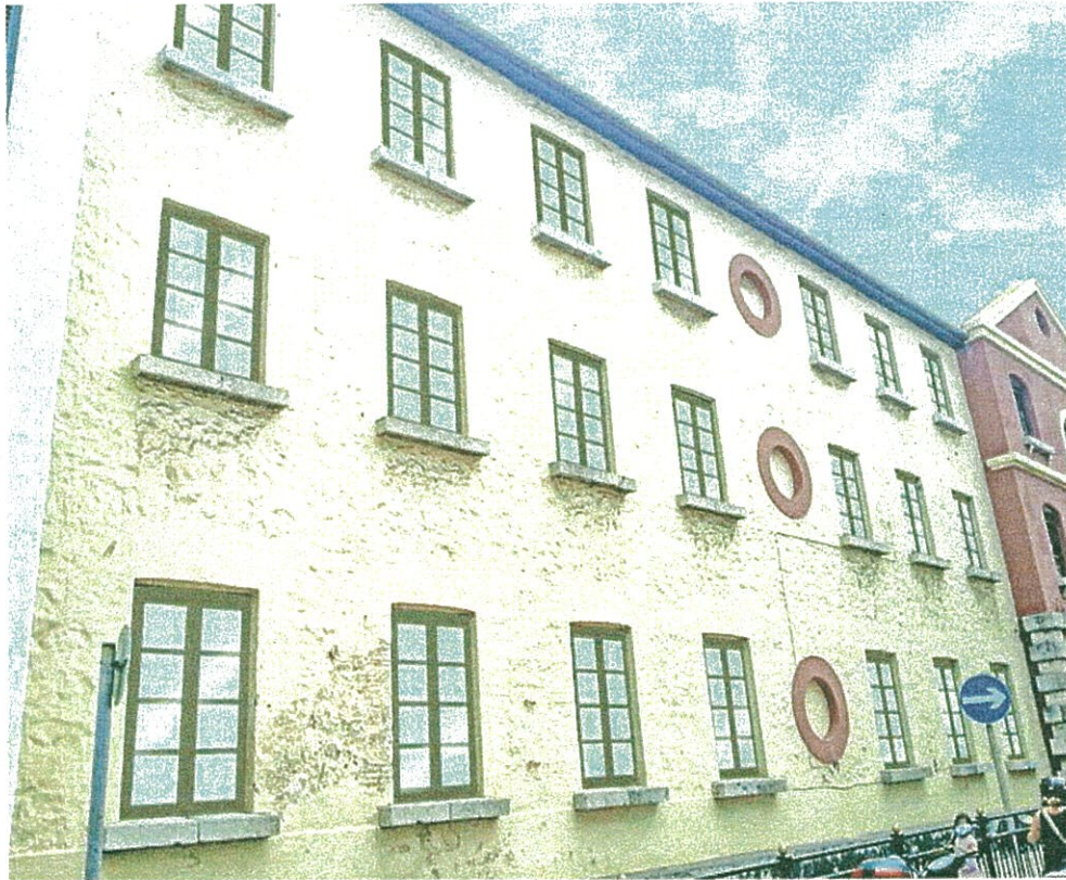
SIDE HUNG INWARD OPENING, TRADITIONAL STYLE TIMBER FRAME WINDOWS AND BEADING WITH A GLOSS PAINT FINISH AND DOUBLE GLAZED UNITS
