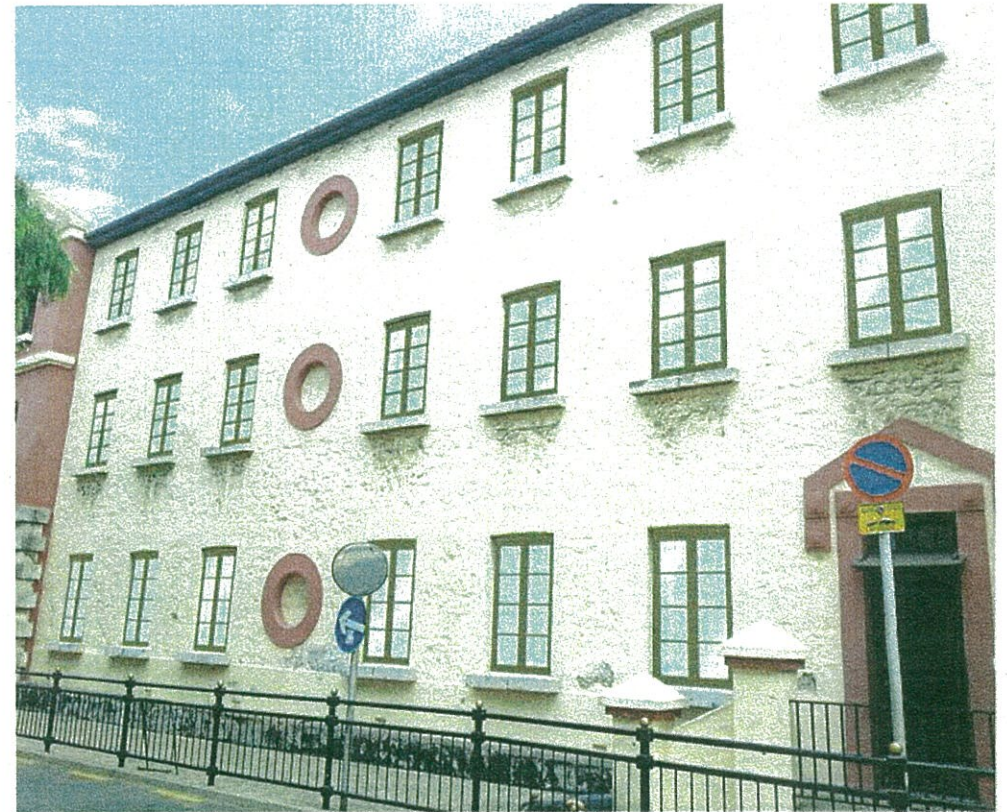
SIDE HUNG INWARD OPENING, TRADITIONAL STYLE TIMBER FRAME WINDOWS AND BEADING WITH A GLOSS PAINT FINISH AND DOUBLE GLAZED UNITS
