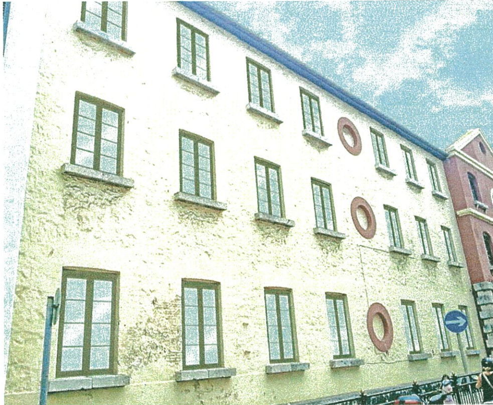
SIDE HUNG INWARD OPENING, TRADITIONAL STYLE TIMBER FRAME WINDOWS WITH A GLOSS PAINT FINISH AND PVC BEADING WITHIN DOUBLE GLAZED UNITS
