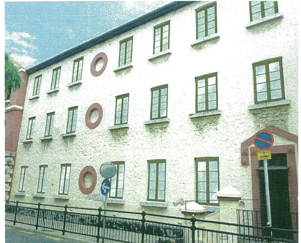
SIDE HUNG INWARD OPENING, TRADITIONAL STYLE TIMBER FRAME WINDOWS WITH A GLOSS PAINT FINISH AND PVC BEADING WITHIN DOUBLE GLAZED UNITS
