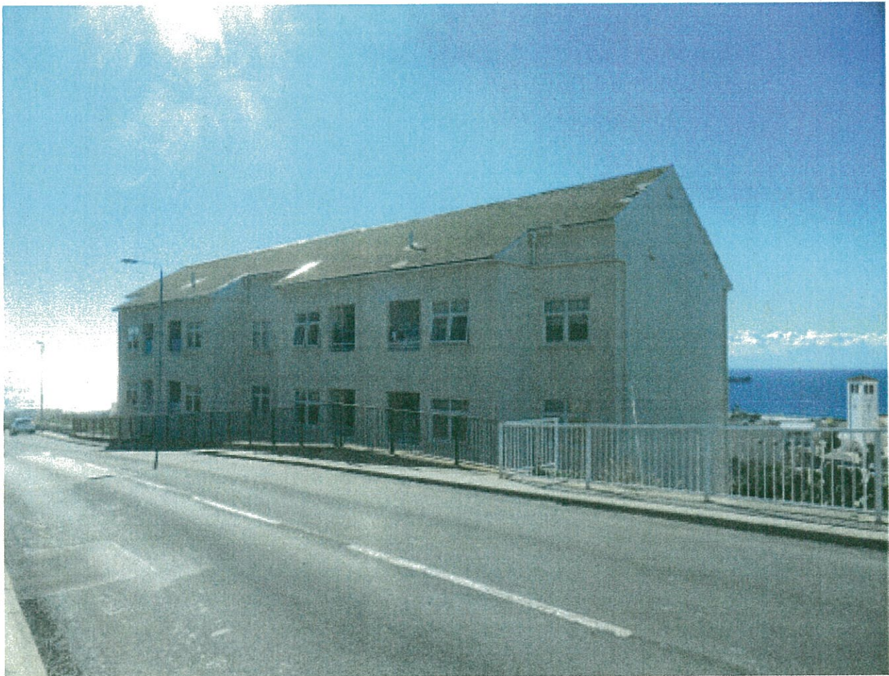
Northeast elevation of building
