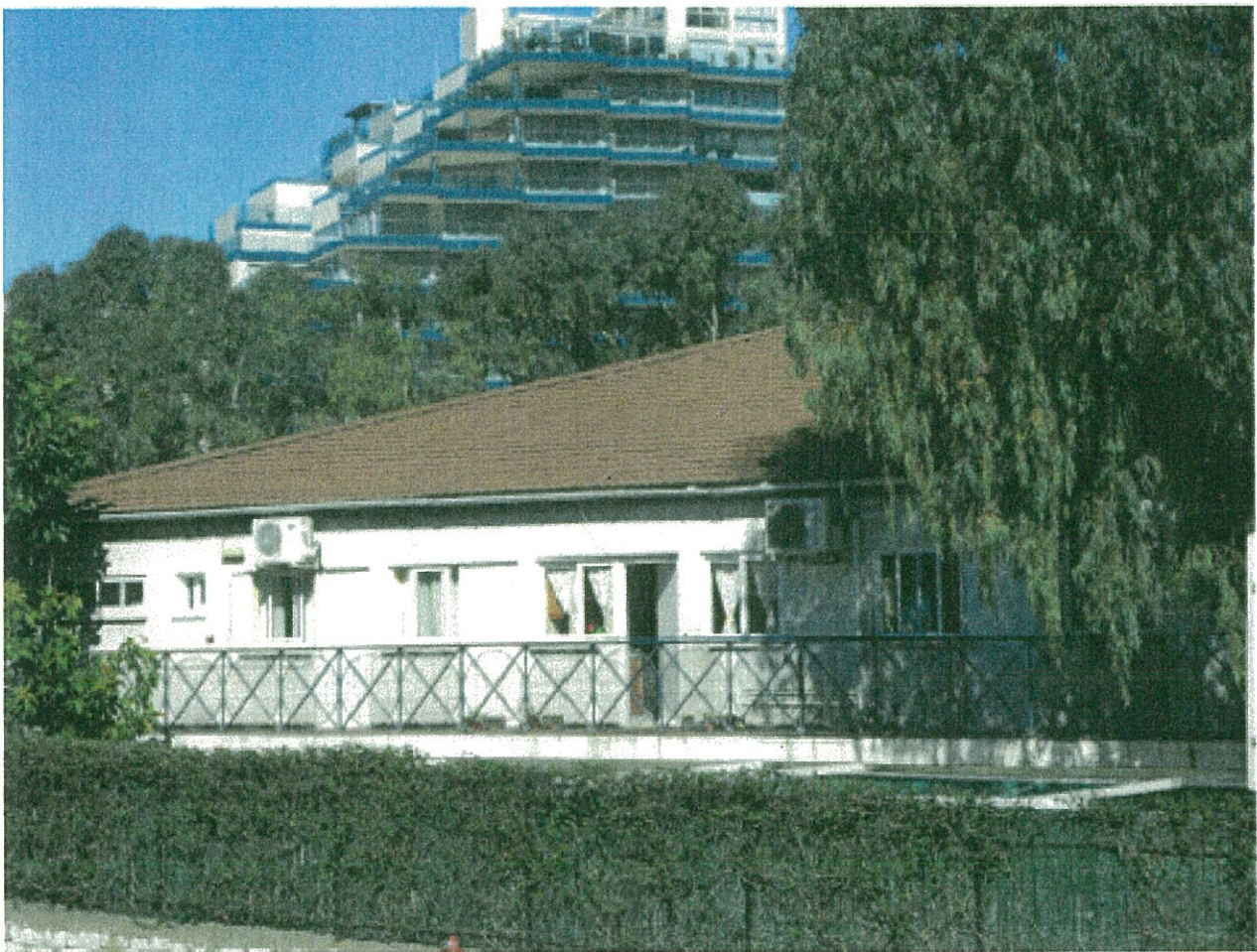
Southeast elevation - note presence of large eucalyptus tree
