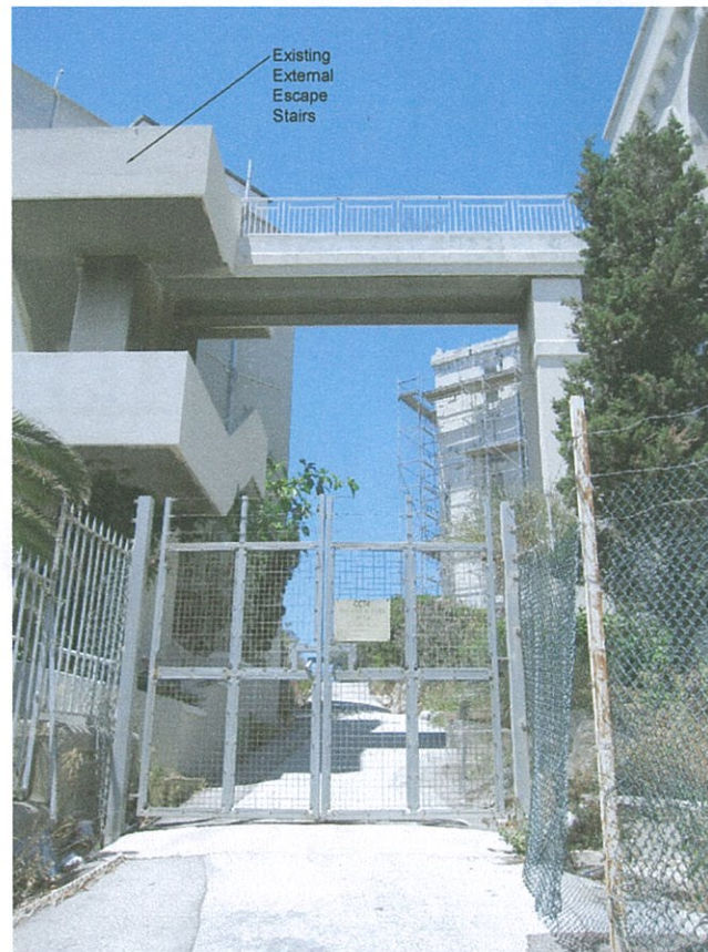
Photo 5: Existing External Escape Stairs
