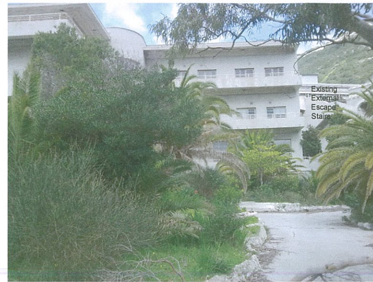
Photo 2: Front of Building and Gardens
