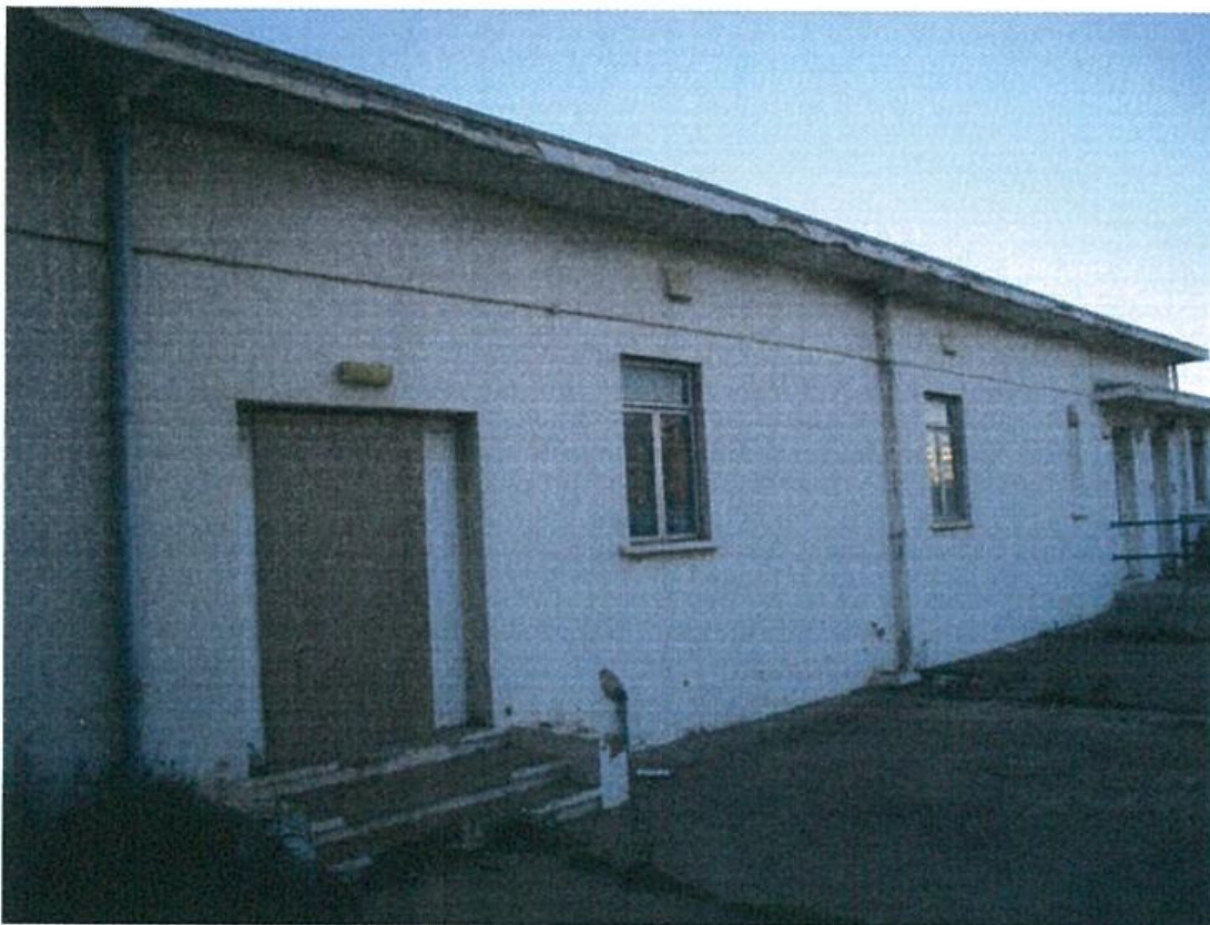
Photograph 2 – North Eastern Elevation of the single storey kitchen area.
