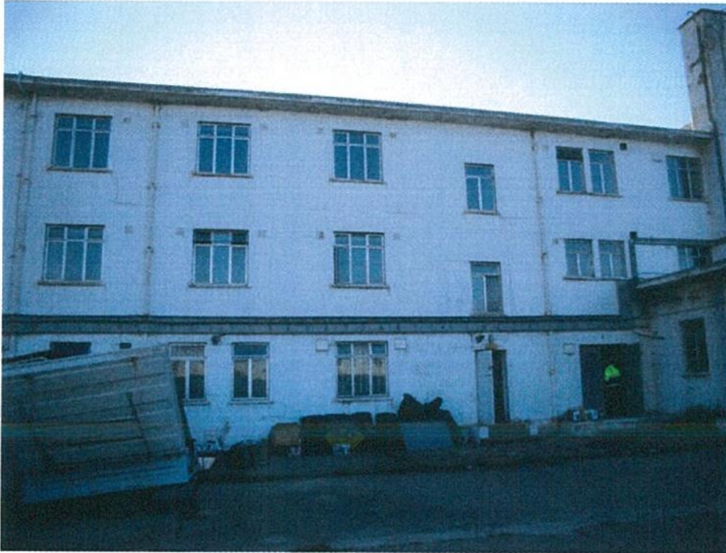
Photograph 1 – North Western Elevation of the three storey accommodation block.
