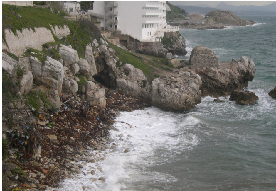
Fig. 6. This area of sector 2 was unfortunately used as a dumping ground and the unstable and contaminated nature of the substrate has negatively affected the intertidal diversity in this part of the sector.
