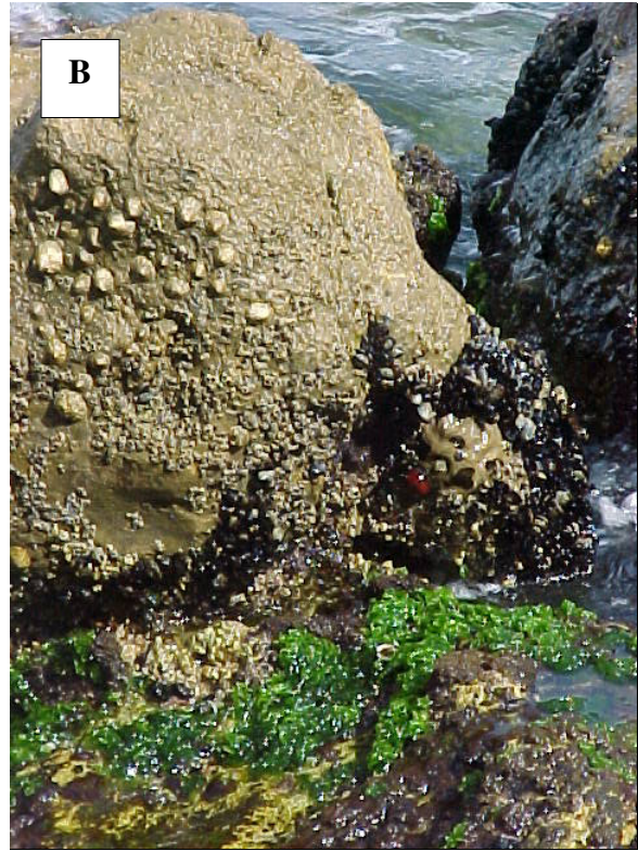
Figs.3 A&B. Sector 1 groynes and rock armoury show evidence of being colonized (A-Eastern Beach, B-Catalan Bay).
