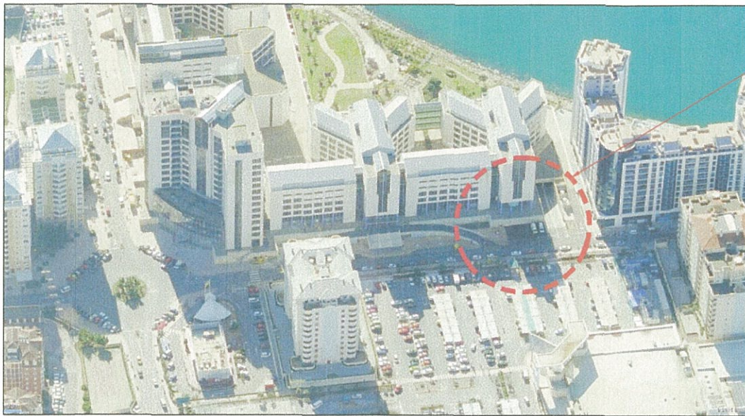
AERIAL VIEW OF SITE
