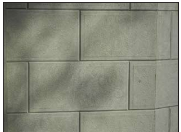
Bevelled edges to this stone cladding results in a more authentic finish
