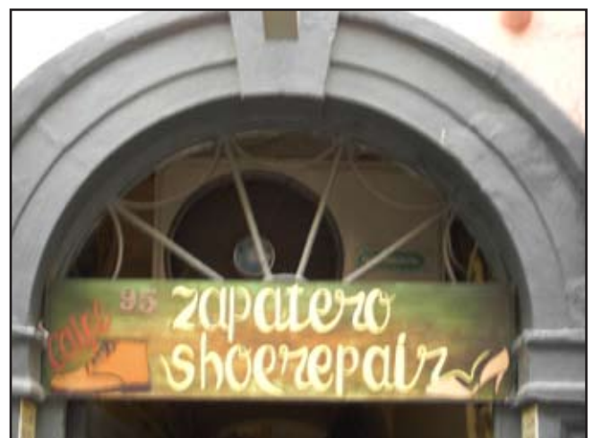
Air condition units concealed behind fanlight.
