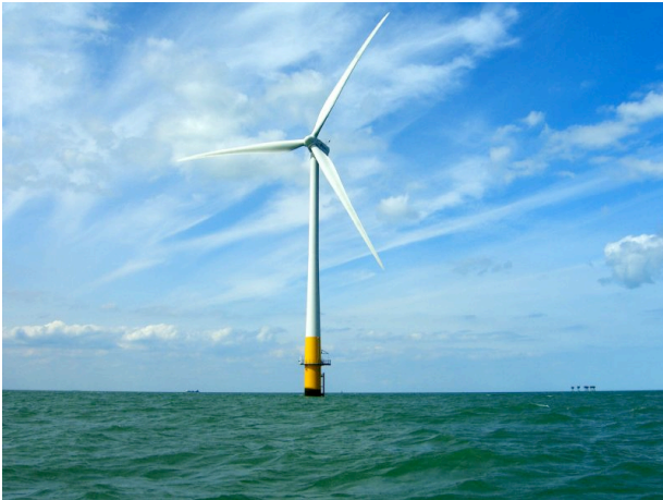
Figure 8: an Offshore Wind Turbine at Blyth 31
