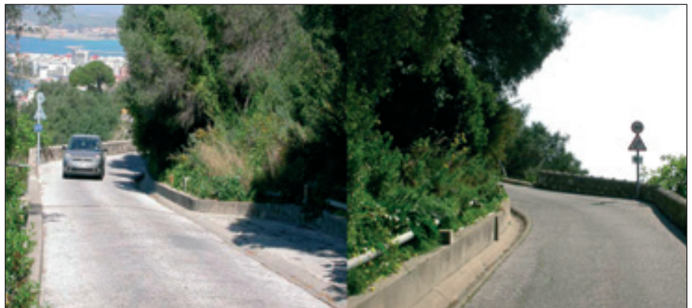
Figure 2. Engineer Road bend, looking north.
