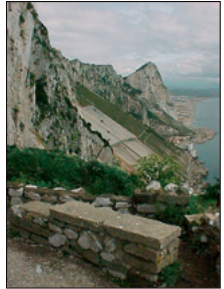
Figure 7. The lookout point that overlooks the eastern side of the Rock is in a state of severe neglect.
