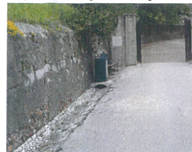
Repairs to existing wall, drainage channel
