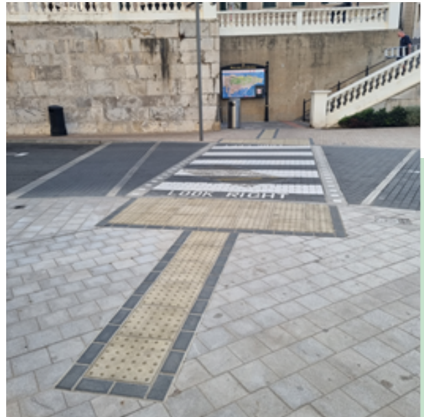
Tactile paving at crossing by British Memorial Steps.
